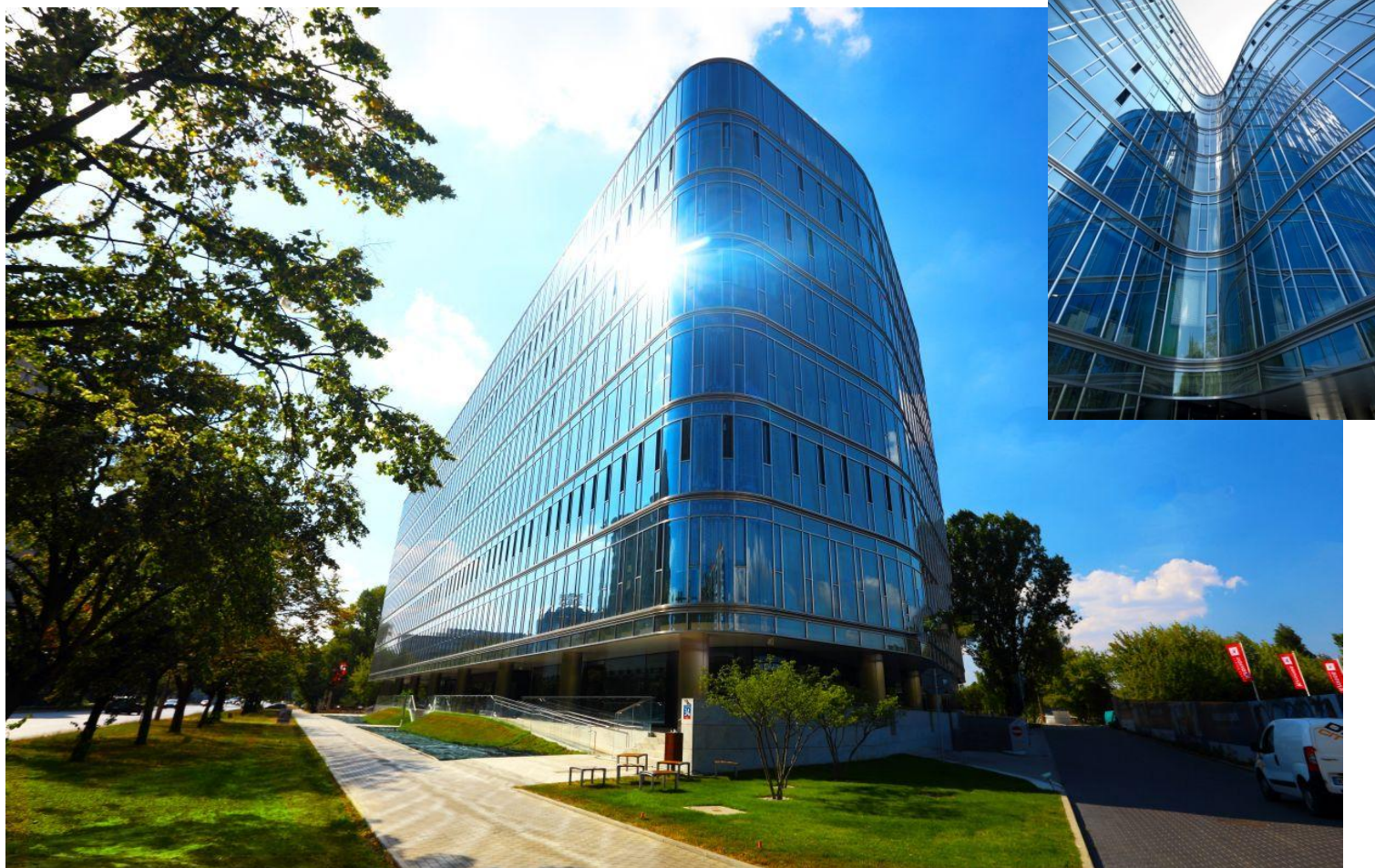
Ambassador Office Building, Warszawa Projekt: AMC Andrzej M. Chołdzyński Sp. z o.o.
