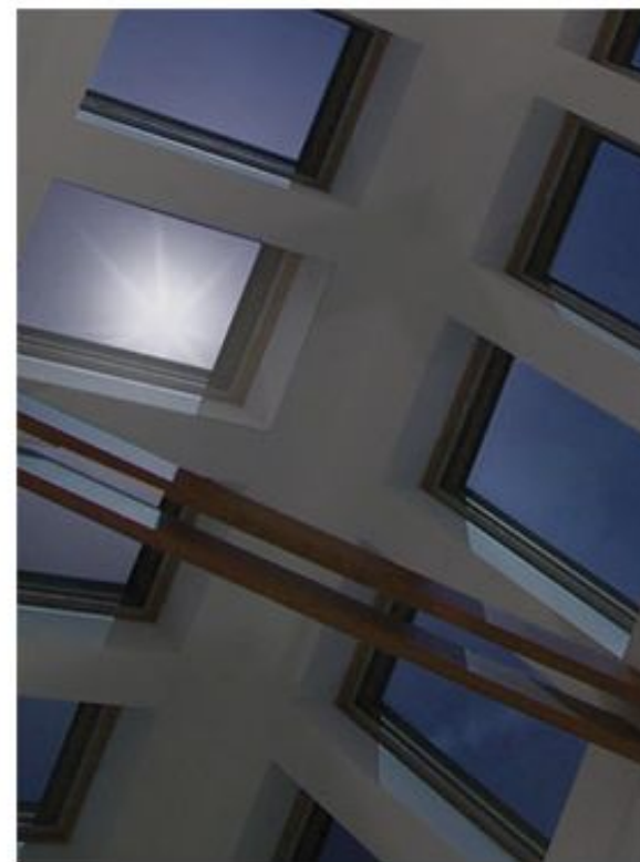
Bridge Street skylights tinted to block the glare and heat.
